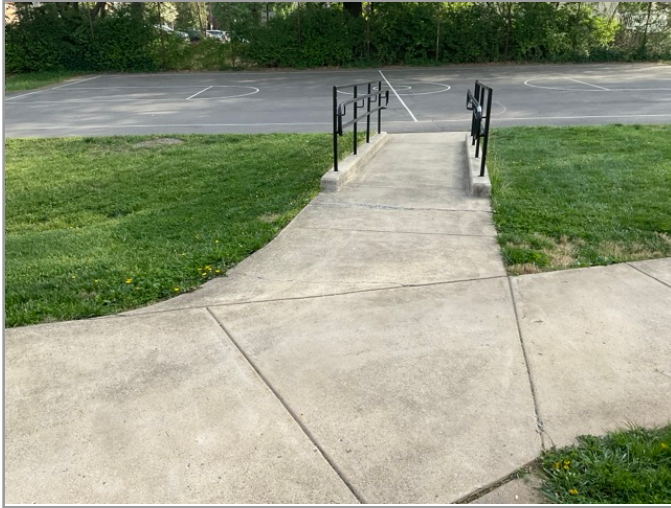
ACCESSIBLE ROUTE TO PLAYGROUND
