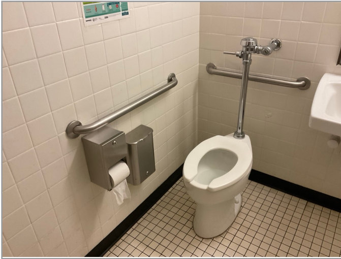
TOILET STALL OVERVIEW
