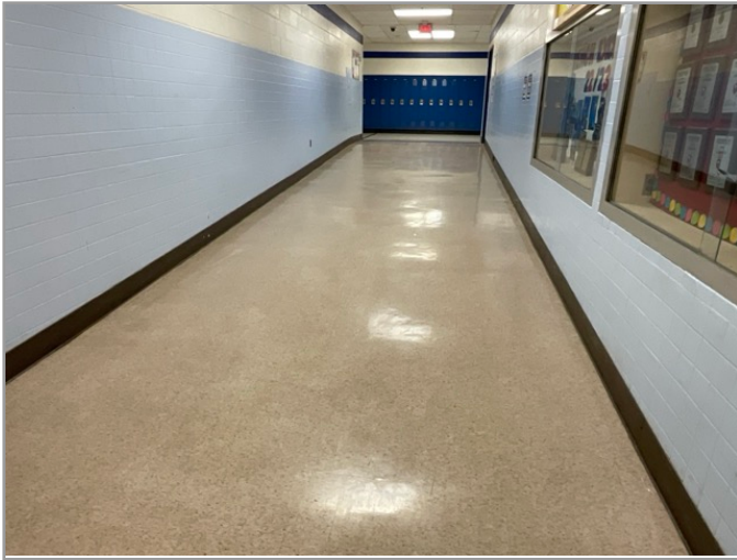
ACCESSIBLE INTERIOR RAMP
