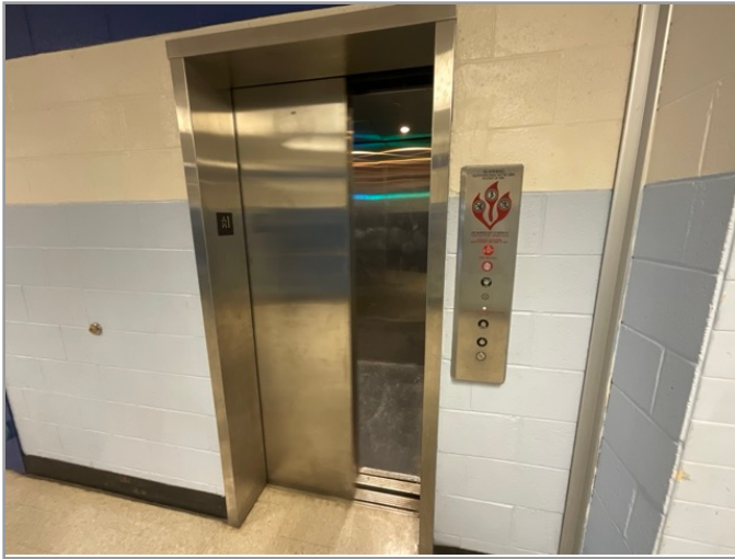
LOBBY LOOKING AT CABS (WITH DOORS OPEN)
